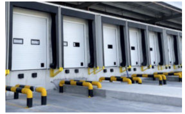
Guide Rail Steers the truck straight into the bay
